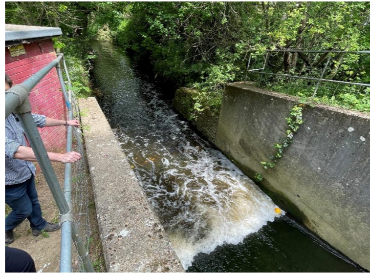
Photo 73: Downstream of Airport Way culvert
