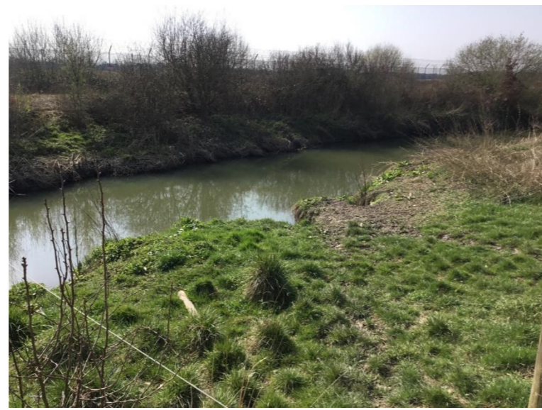
Photo 14: Towards end of straightened section of River Mole, wide and steep banks
