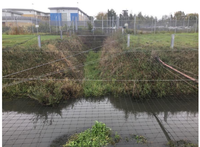
Photo 103: Concrete outfall and vegetated spillway
