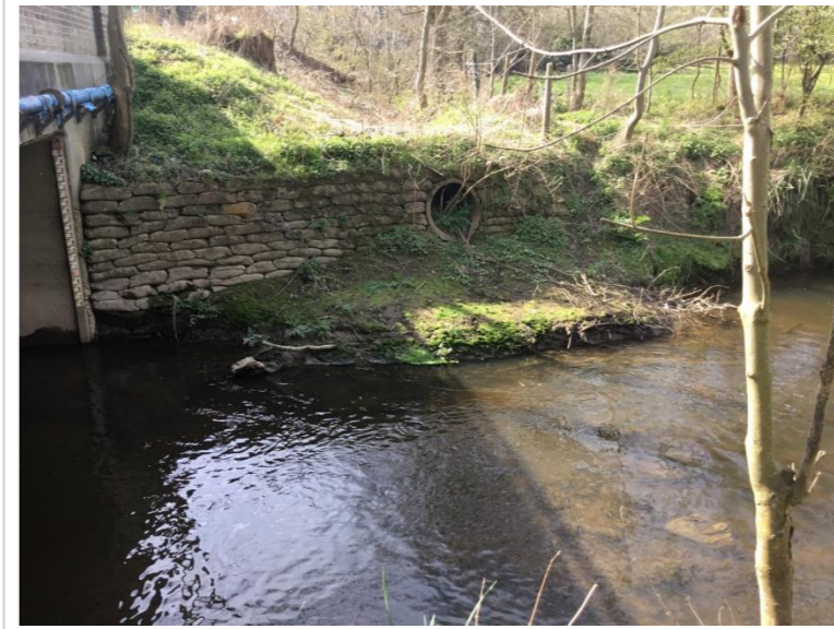
Photo 39: Dry ditch outfall on left bank immediately downstream of Brighton Road bridge
