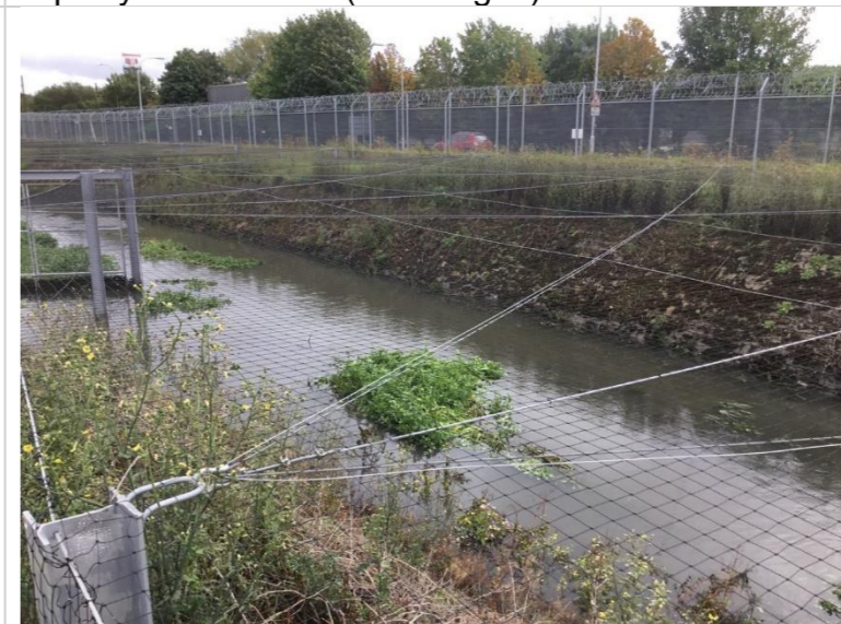
Photo 93: Concrete blockwork on left bank and mid channel vegetated bars
