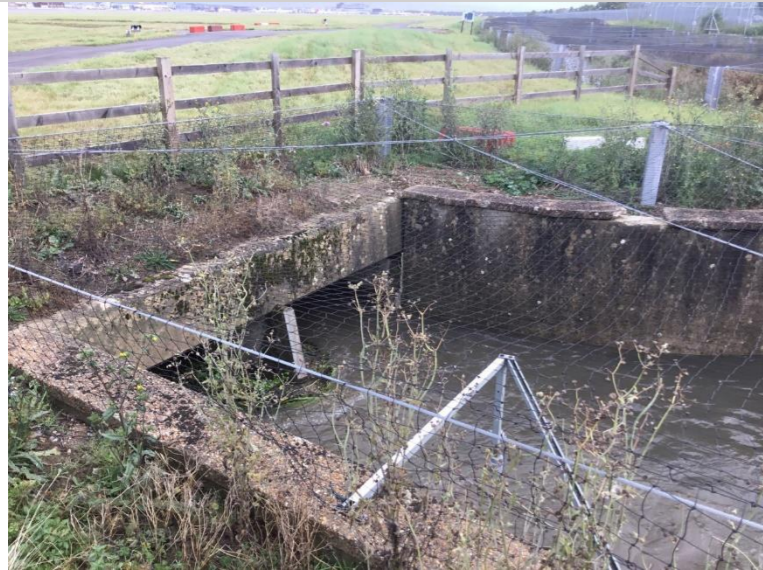
Photo 7: Runway box culvert inlet and divider wall
