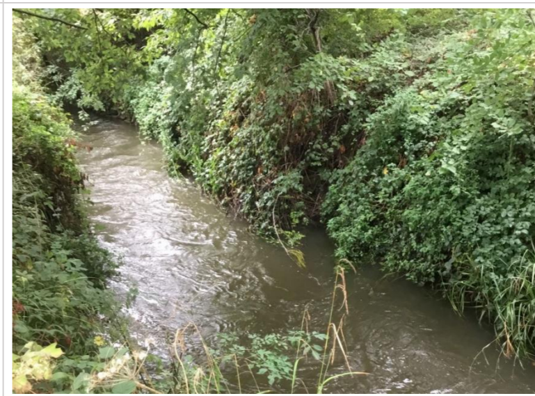
Photo 65: Vertical heavily vegetated banks approaching South Terminal
