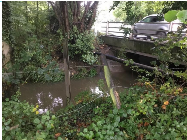
Photo 44: Radford Road bridge at furthest upstream extent
