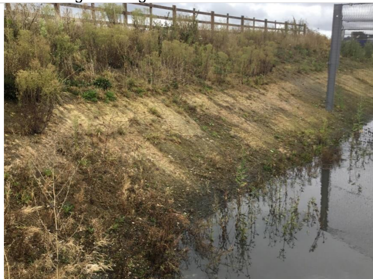
Photo 91: Geotextile over clay banks exposed
