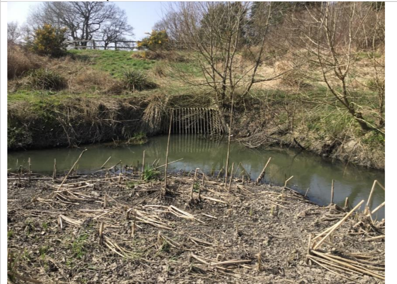
Photo 18: Culvert outfall from Westfield Stream on left bank
