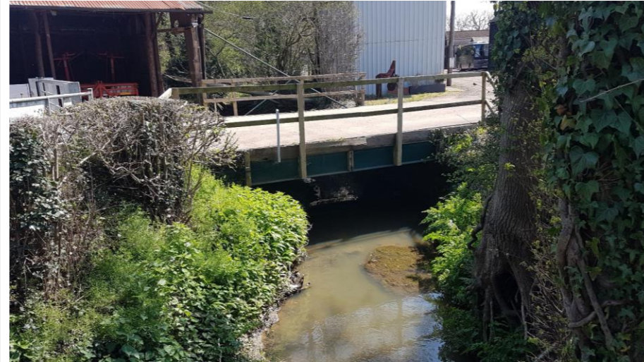
Photo 130: Road bridge set into vertical bank face
