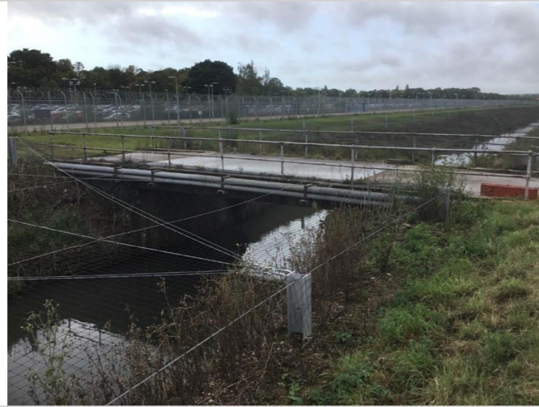
Photo 107: Access bridge and concrete abutments
