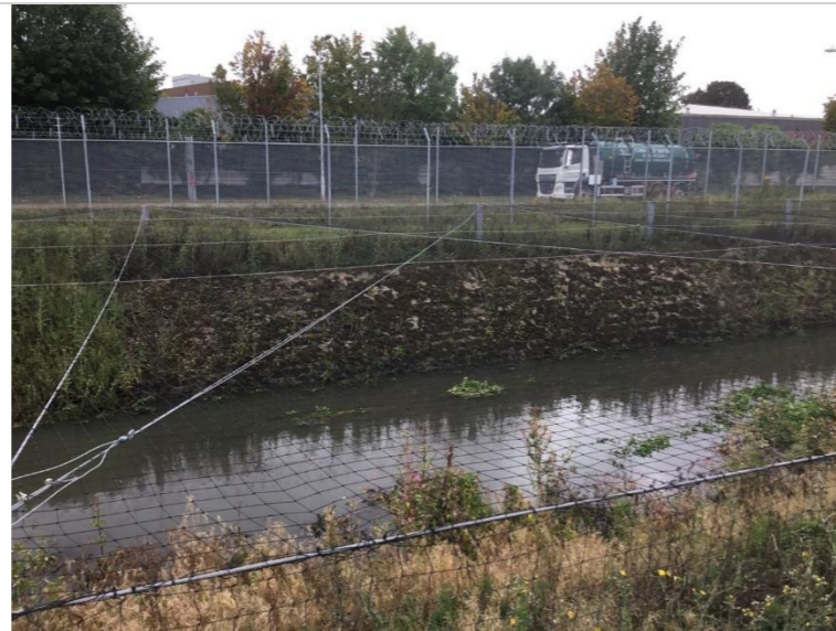
Photo 89: Concrete blockwork bank exposed on left bank
