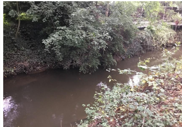
Photo 82: Bank protection including wooden slats and gabion baskets on right bank as bank protection adjacent residential area (right of image)
