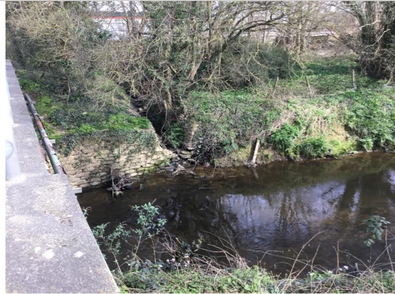
Photo 37: Ditch outfall on right bank immediately upstream of Brighton Road bridge
