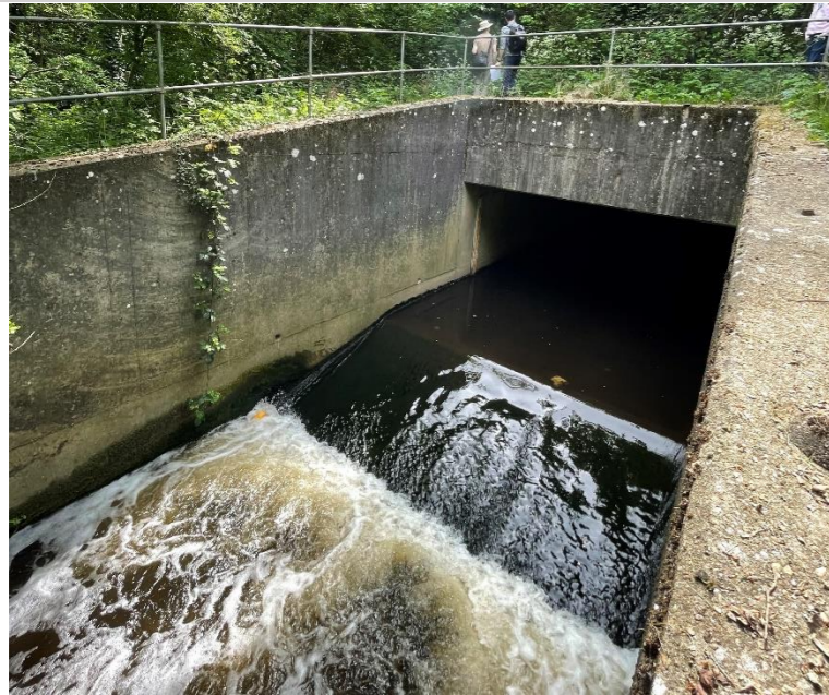
Photo 72: Airport Way culvert outlet and weir structure
