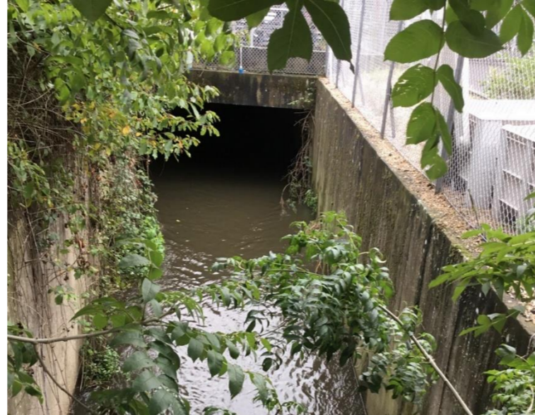
Photo 67: South Terminal culvert inlet
