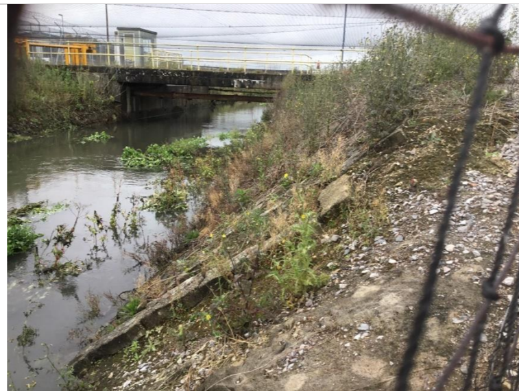
Photo 92: Concrete blockwork on right bank
