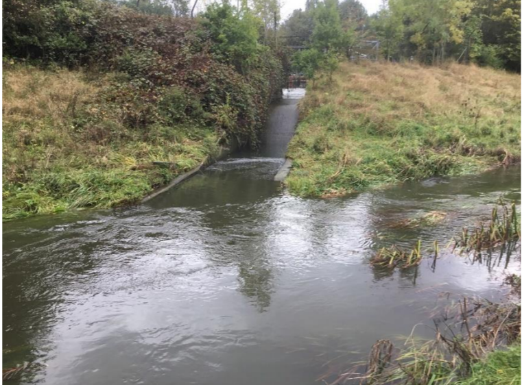
Photo 29: Concrete outfall from Pond D
