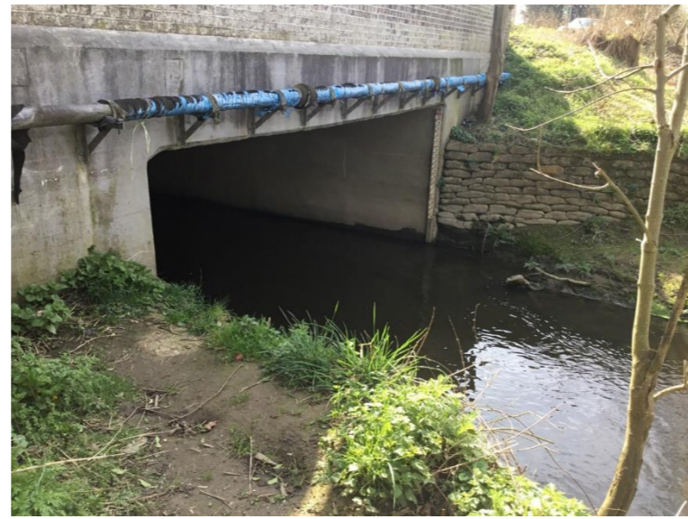
Photo 38: Downstream side of Brighton Road bridge
