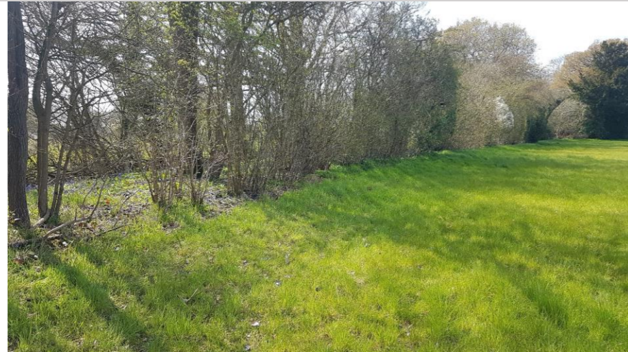
Photo 135: Left bank top and low embankment bordering watercourse and meadow
