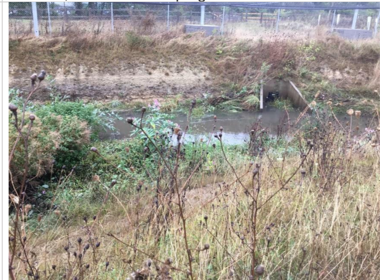
Photo 52: Outfall with concrete headwall on right bank
